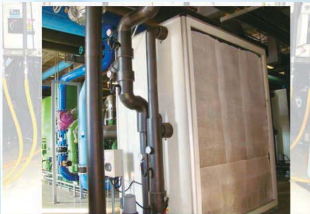
FFU pre-filter拆除前
