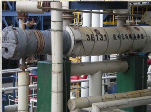
酸水氣提塔(3C130)再沸器(3E131)改出自產低壓蒸氣
