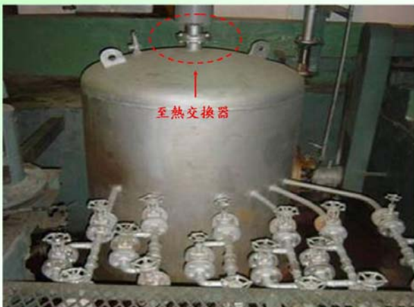
M/C#1烘缸冷凝水槽尾汽回收熱交換改善
